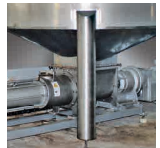
Feed process in a KL100RL120-8 V4A progressing cavity pump
